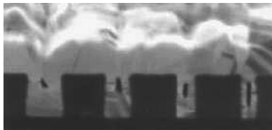
Fig. 1. An image of copper deposited from electrolyte. Voids are apparent in the trenches. The picture is taken from [29].
